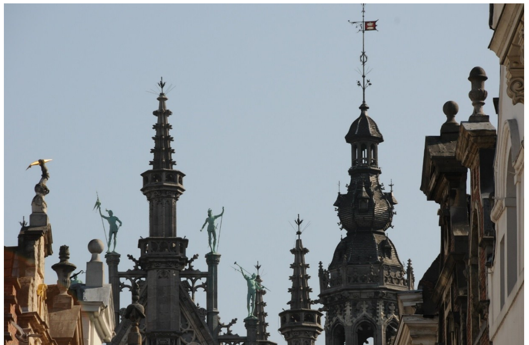
Rooftop ornaments As seen from Grand Place M. Vanhulst © urban.brussels
