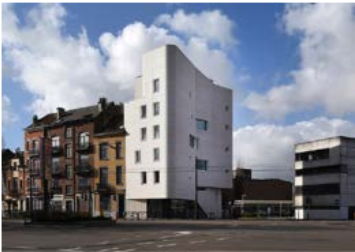
REF: Navez House, V+ & MSA, Schaerbeek
