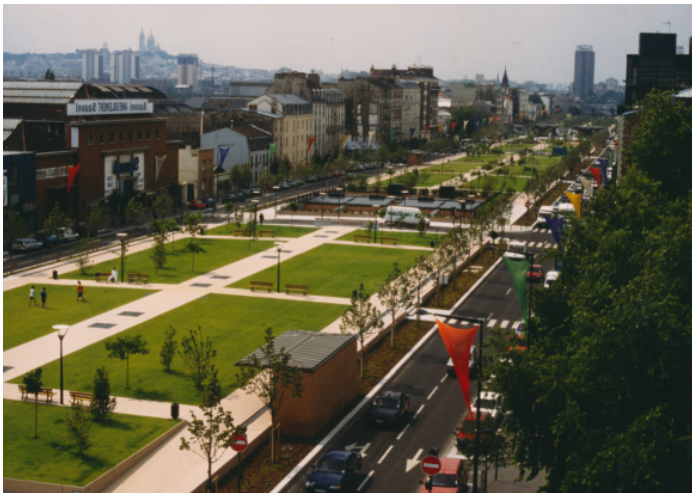
REF: Couverture de l'autoroute A1, Paris, France
