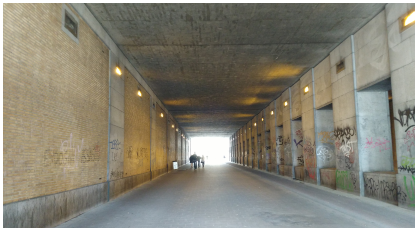
Tunnel Nord © Google Maps
