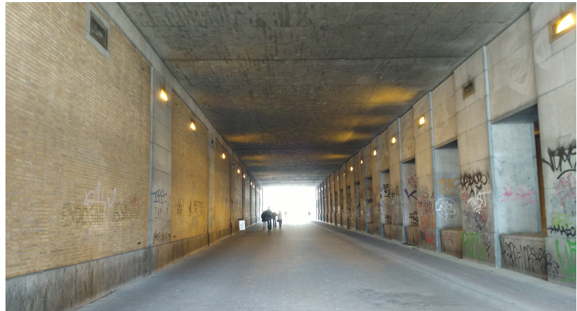
Noordtunnel © Google Maps
