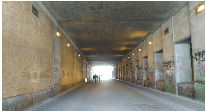
Tunnel Nord © Google Maps
