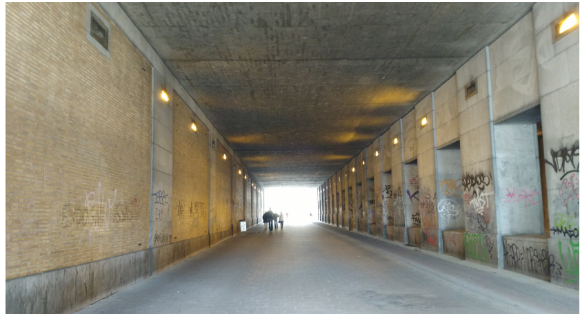
Noordtunnel © Google Maps
