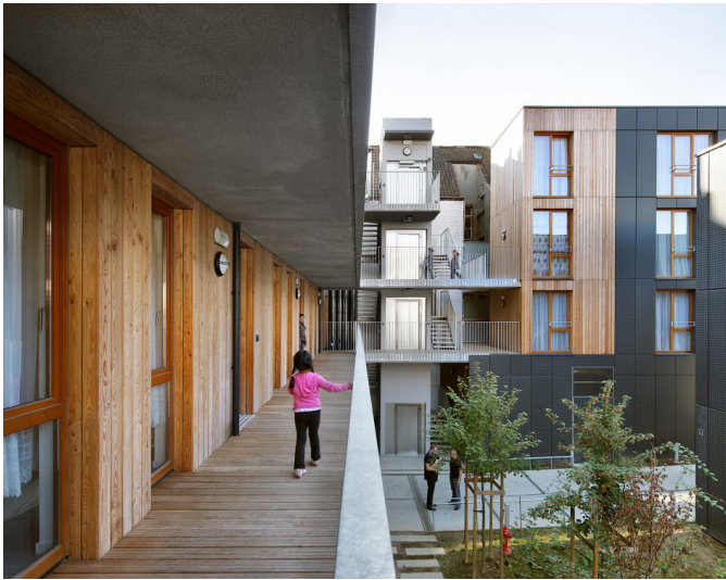
Savonnerie Heymans, Brussel, MDW Architecture
