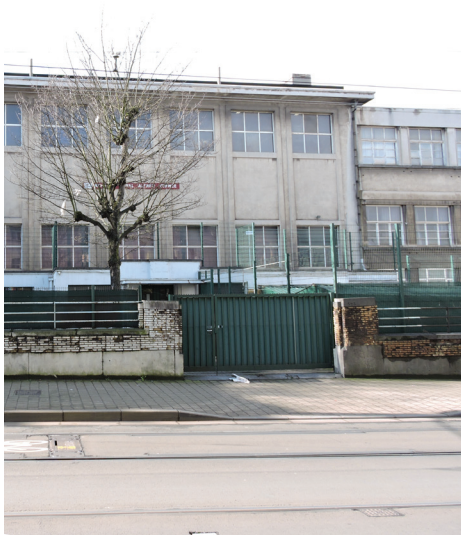
Ecole "les griottes" - chaussée de Haecht
